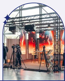
TRUSSING FOR LIGHTING AND OVERHEAD FITTINGS
